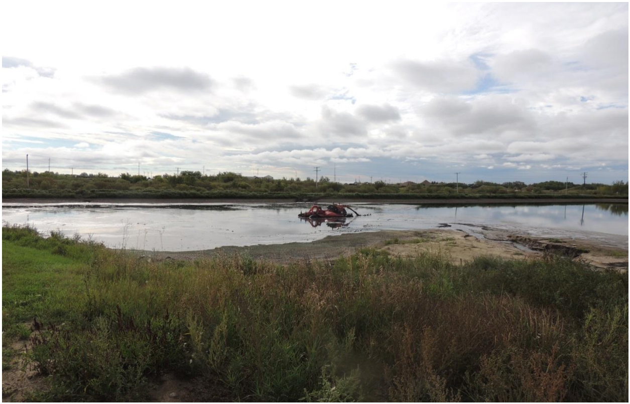
Agitating Sludge in Lagoon to Facilitate Pumping
