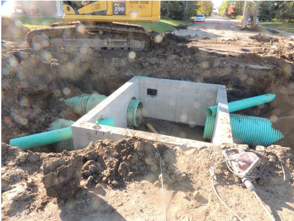
Storm Main Installation Typical Manhole 2016
