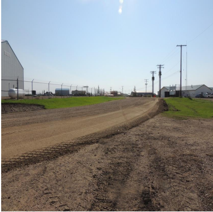
Industrial Area Road Improvements Traffic Gravel 2016
