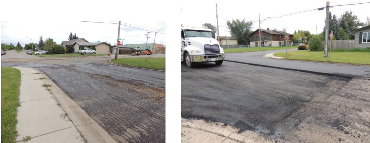
Center St and King St, at 9 th Ave – Asphalt milled, 2016
