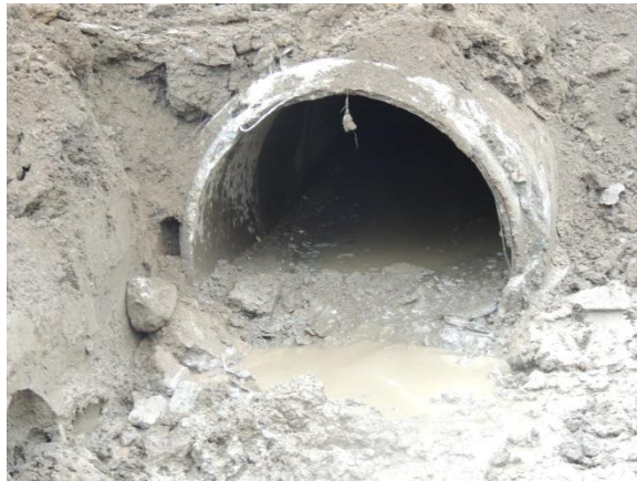
Storm Main Renewal 6 th Ave W – Pipe in poor condition with reduced capacity.
