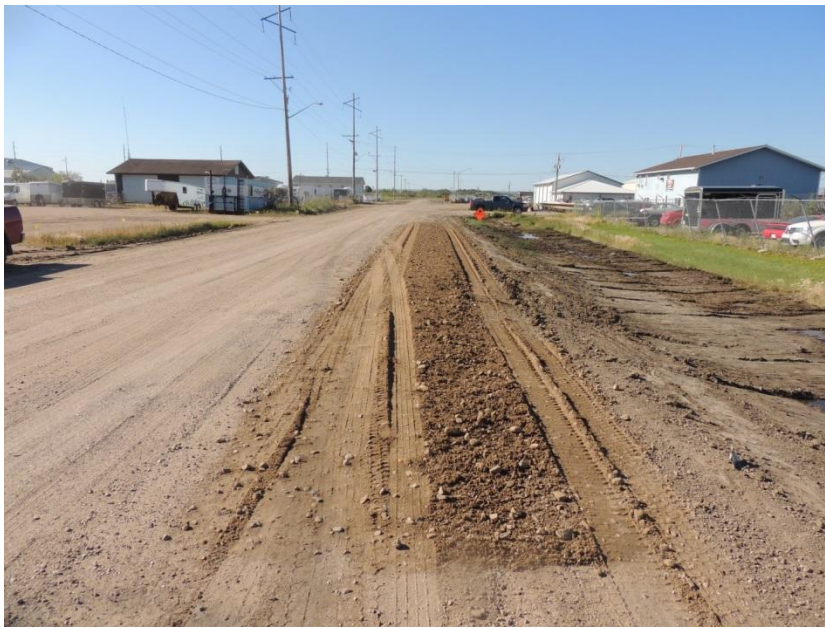
Industrial Area Ditch Improvements and 3" Crushed Pit Run Base
