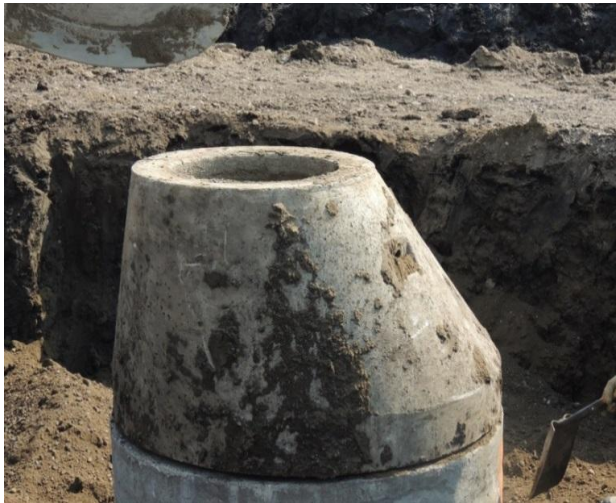
2016 Raising Sanitary Sewer Manholes West Service Road
