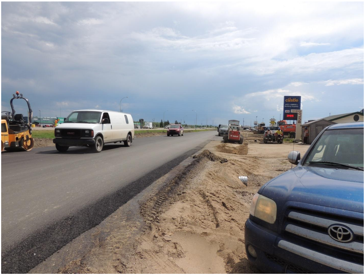
West Service Road in use July 2016
