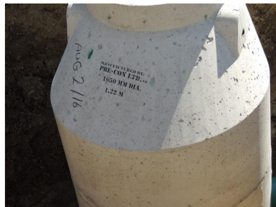
Renew Manhole at the Intersection of Cochin Ave and 4 th St W. (Old manhole had no base)
