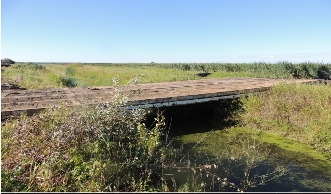
2016 Access Bridge Across the Drainage Channel to Access Cattail Pond (Temporary)
