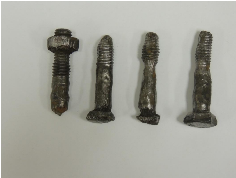
Sample of bolts from the bottom flange of the hydrant removed from 218 8 th St. West. Bolts are steel, not stainless steel.
