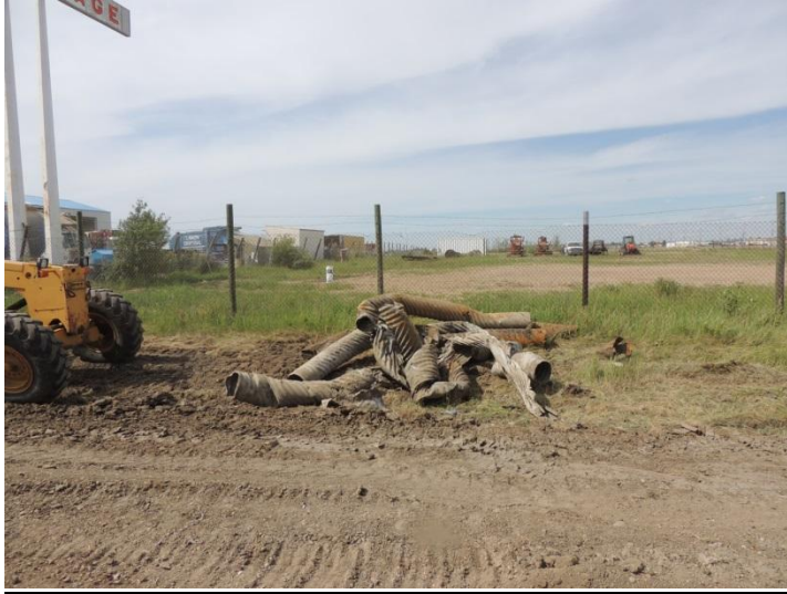
Culverts Removed From Industrial Area 2016
