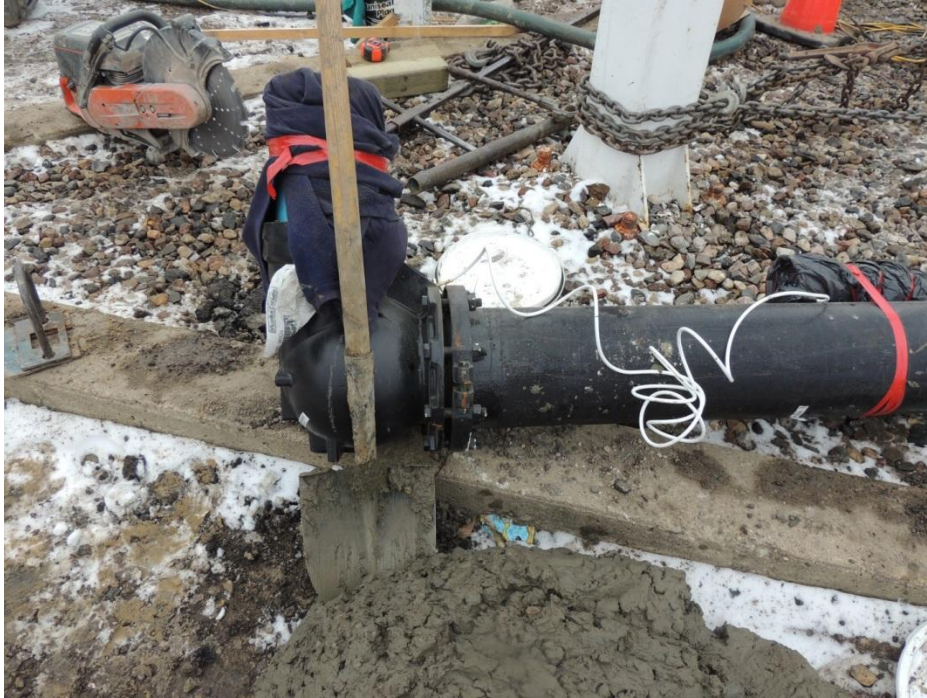
New Hydrant and Anode at 218 9 th St. West November, 2016 ( Fas Gas )
