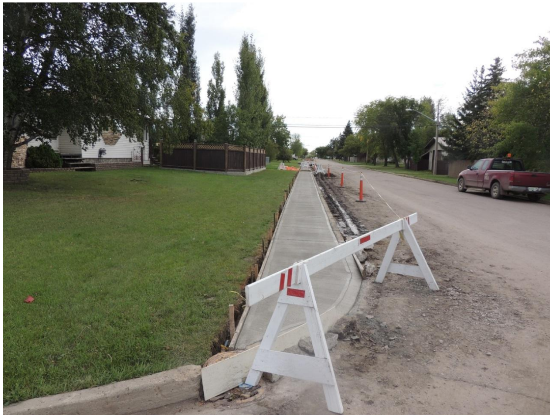
2016 New Sidewalk Under Construction
