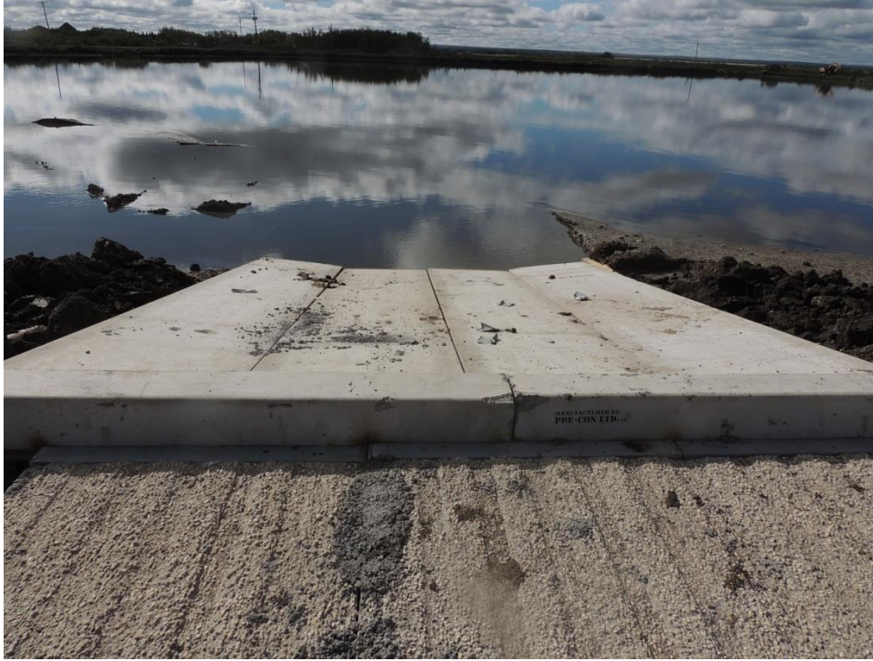
2016 New Concrete Dump Chute Under Construction
