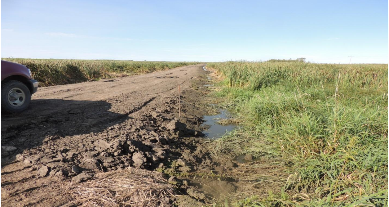
Berm Constructed Across the Cattail Pond
