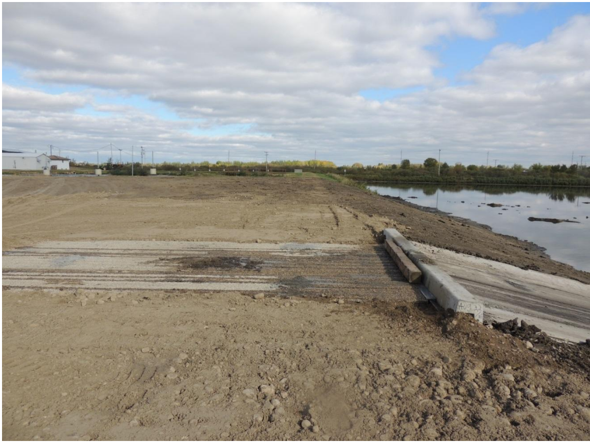
2016 Repaired Berm and New Concrete Dump Chute
