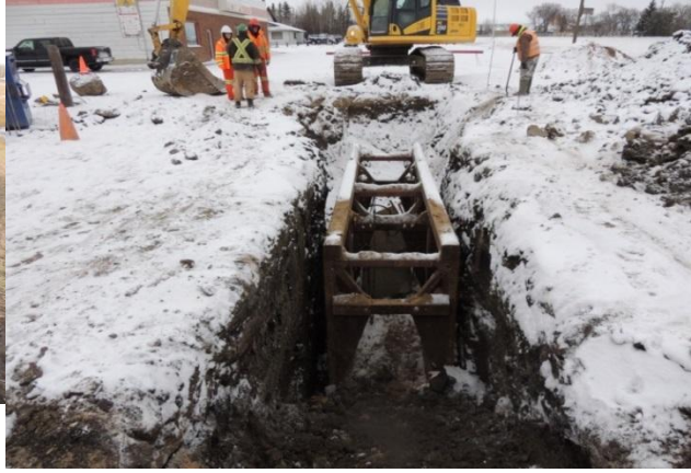
Water Line Installation
