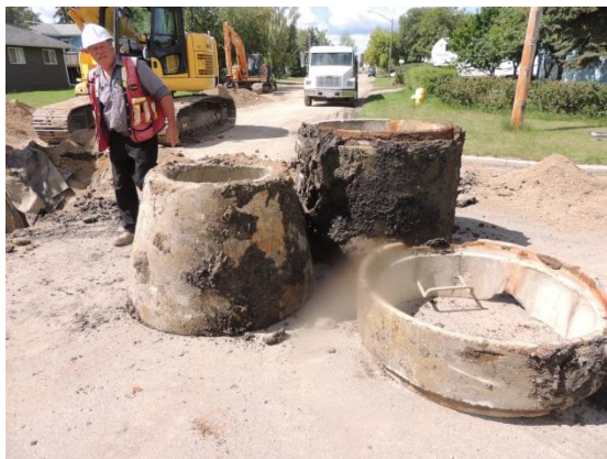
Renew Manhole at the Intersection of Cochin Ave and 4 th St W. (Old manhole had no base)
