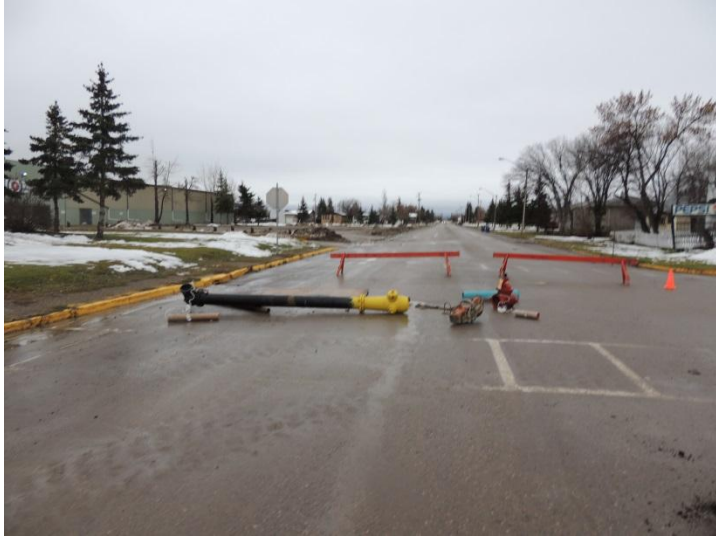
New Fire Hydrant Prepared for Installation at 3 rd St. E November 2016
