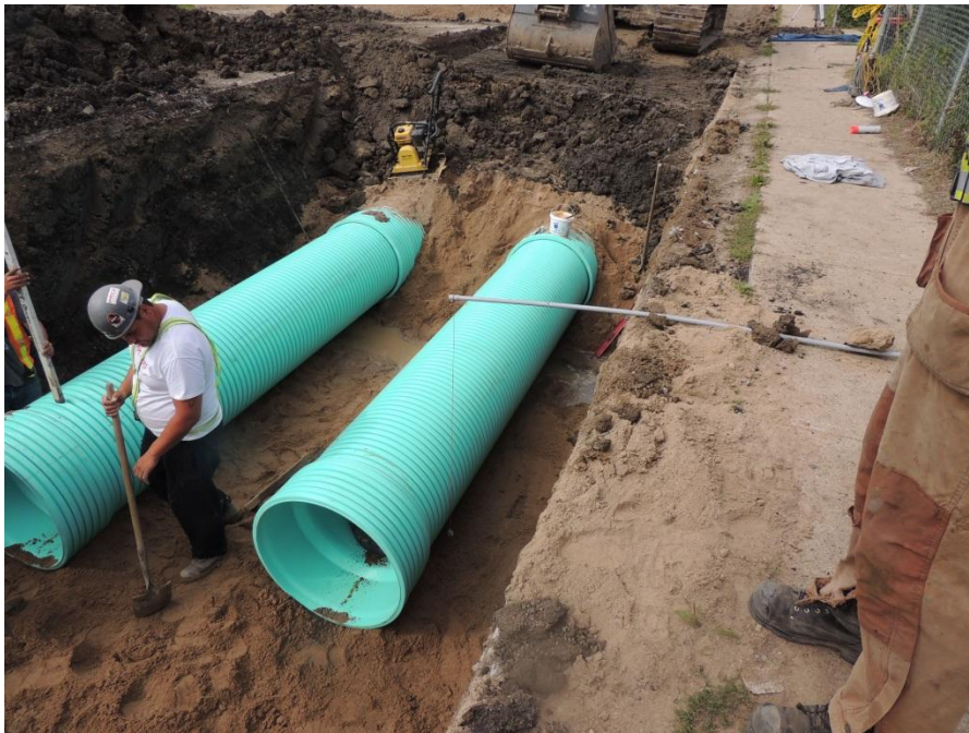
Twin Storm Main Installation 6 th Ave W 2016
