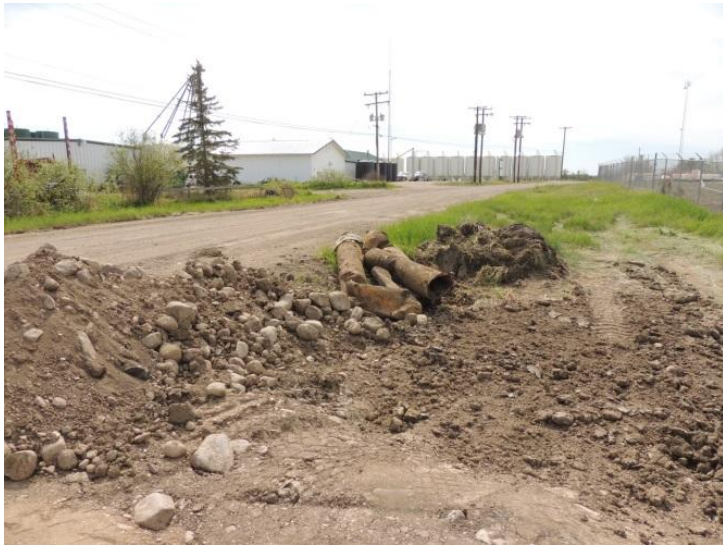
2016 Culverts(Welded Hot Water Tanks) Removed From Industrial Area
