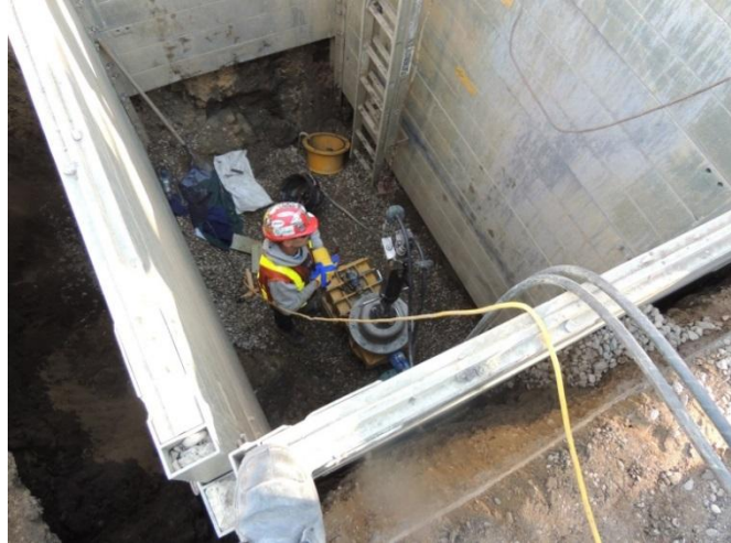
Hot Tapping Water Main Valves – 7 th Ave W and 3 rd St. W 2016
