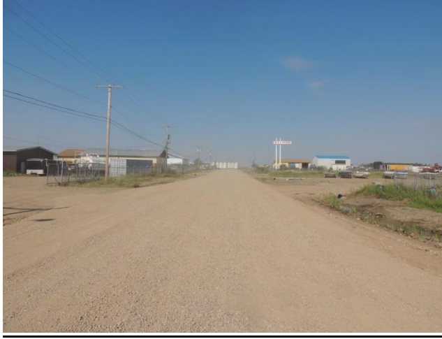
2016 Industrial Area New Culverts, Gravel and Grading
